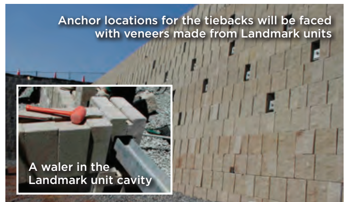
Installation of the tiebacks
