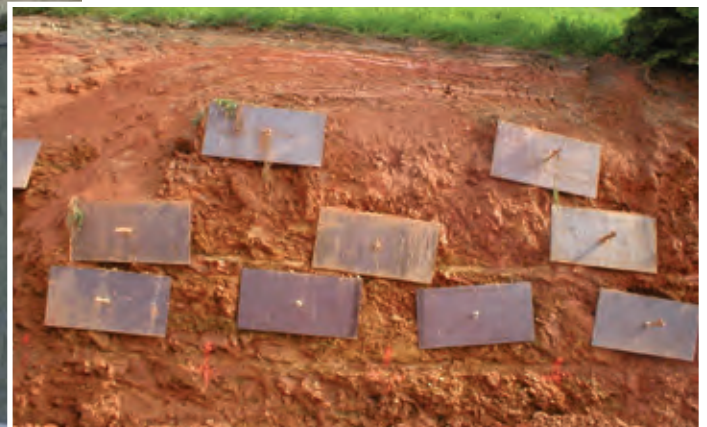
By using soil nails and the Landmark® system, this parking lot was enlarged to meet the developer's needs. The cut was close to a highway, and there was no room to excavate for reinforcement.
