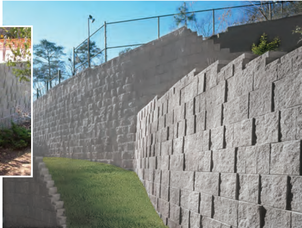
The timbers facing the wall below a tennis court had failed. The owner wanted the wall repaired while the tennis court was in use. By using the Landmark direct-anchorage system, the wall was refaced, and play was uninterrupted.
