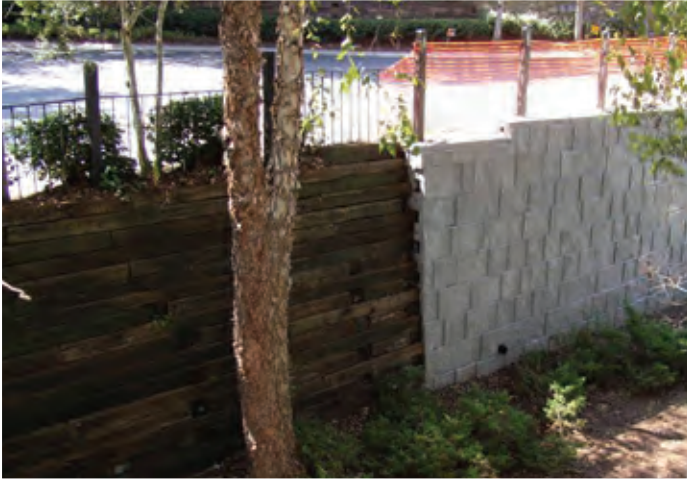
The timbers facing the wall below a tennis court had failed. The owner wanted the wall repaired while the tennis court was in use. By using the Landmark direct-anchorage system, the wall was refaced, and play was uninterrupted.
