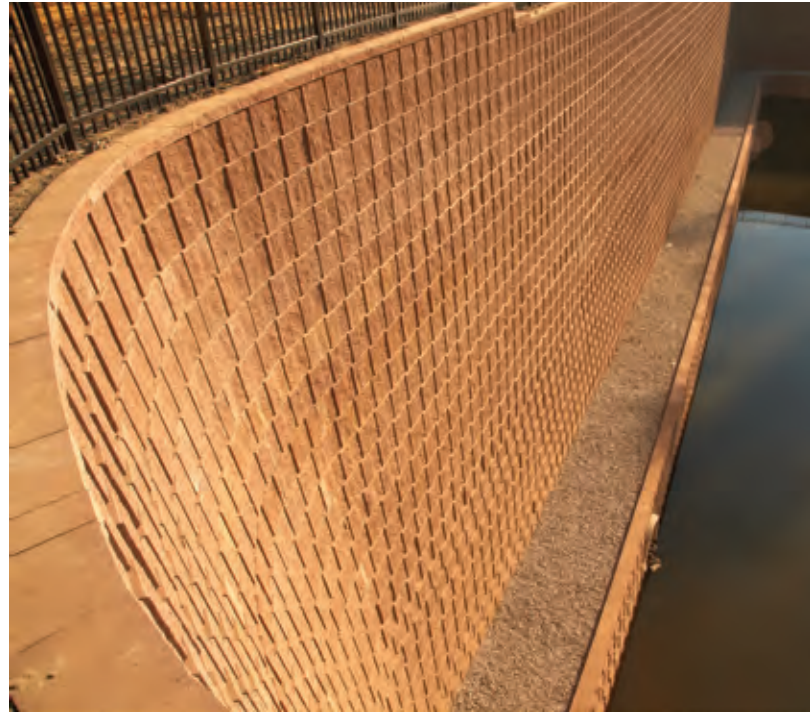
The aesthetics of the Landmark retaining wall system and the nearly vertical system batter were both needed by the designers of this retention pond near a high-profile shopping area.
