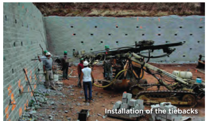
Anchor locations for the tiebacks will be faced with veneers made from Landmark units
