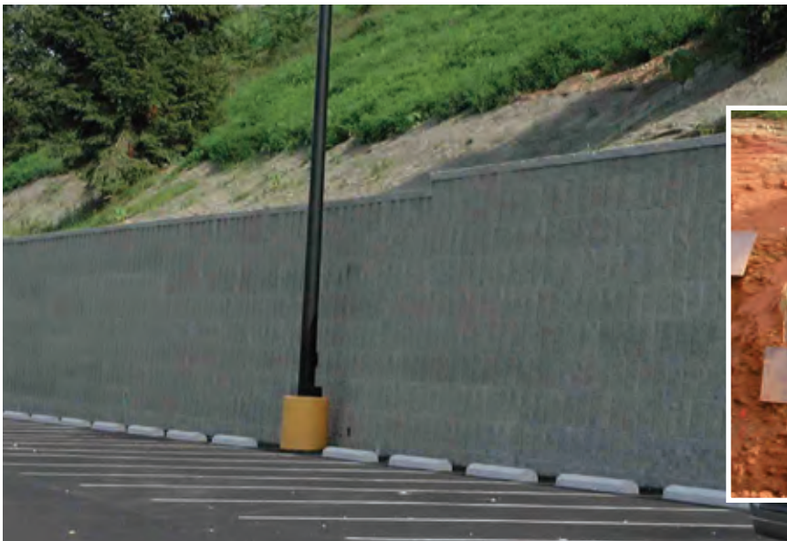
By using soil nails and the Landmark® system, this parking lot was enlarged to meet the developer's needs. The cut was close to a highway, and there was no room to excavate for reinforcement.
